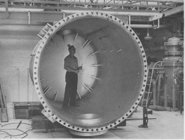
SHELL OF HEATER for new hypersonic wind tunnel facility is checked by designer John C. Weydert (7133). Steel shell, 92 in. in diameter, will be up-ended into a pit and packed inside with 14 in. of insulation material. Some 25,000 lbs.
